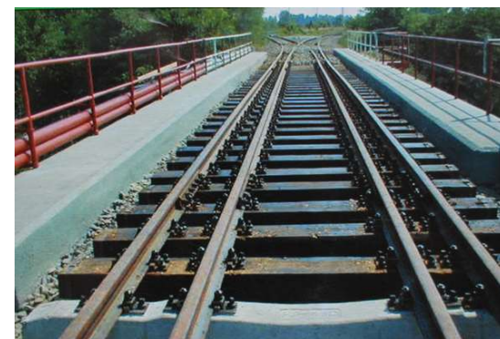
Dual Gauge (1435mm-1520 mm); Railway Track on the Hungary-Ukraine Border ( source: internet )
